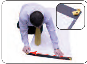
Apply the hanger to the top inside edge of the panel ensuring that it is flush to the panel edge.
