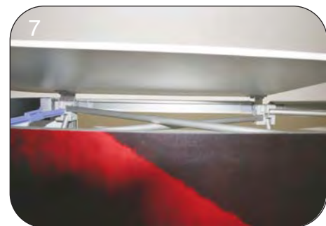
7-8. Install counter tops ensuring aluminium brackets insert securely into hubs.
