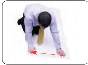
Remove the backing paper from the kicker and apply it to the bottom edge of the panel.
